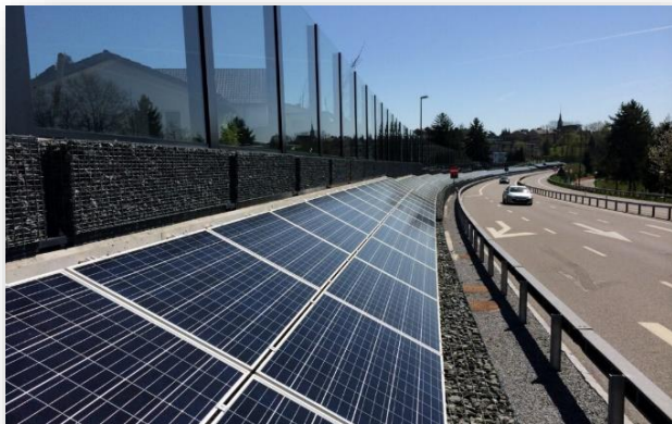
Solarpanels an Autobahnen
